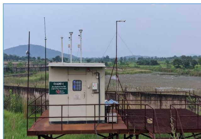
CAAQMS-4 Near Railway Siding
