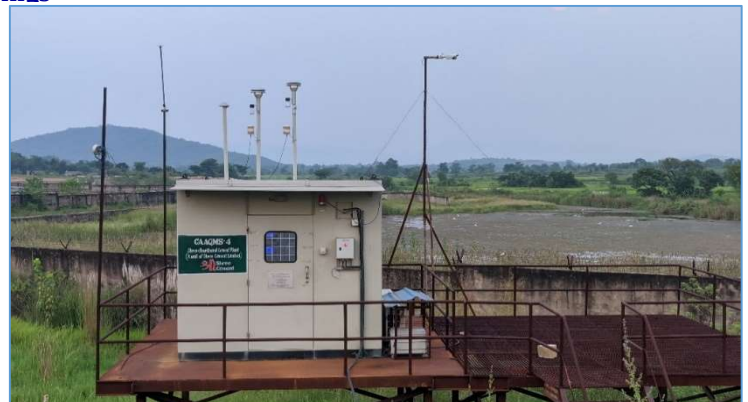
CAAQMS-3 Near Railway Siding
