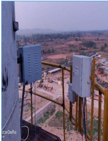
Opacity meter installed at Cement Mill Stack
